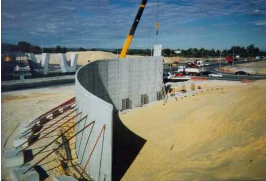
Figure 11. Panels Erected and temporarily propped in position.
