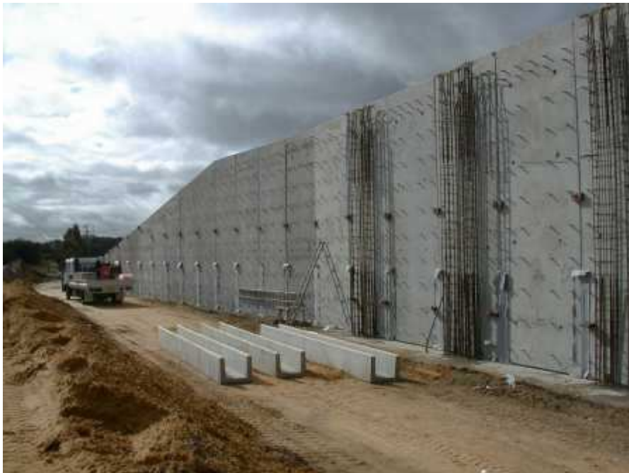
Figure 12. Column reinforcement in position ready for channel forms.
