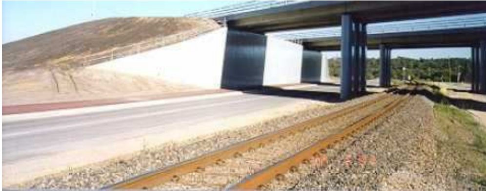
Figure 13. Completed Abutment wall with SWMR in foreground.
