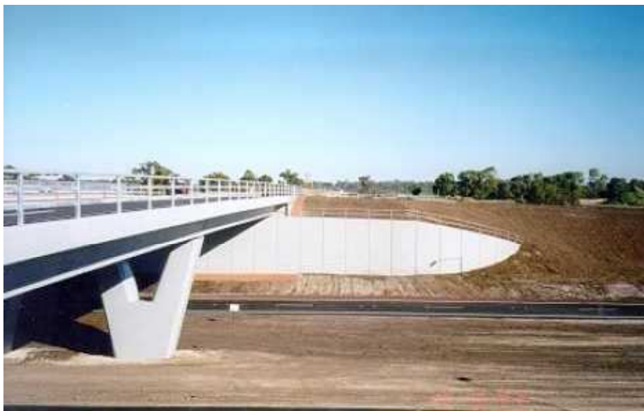
Figure 14. Front View of Completed Abutment
